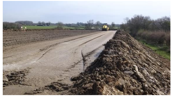
Image showing the development of the trial embankment
