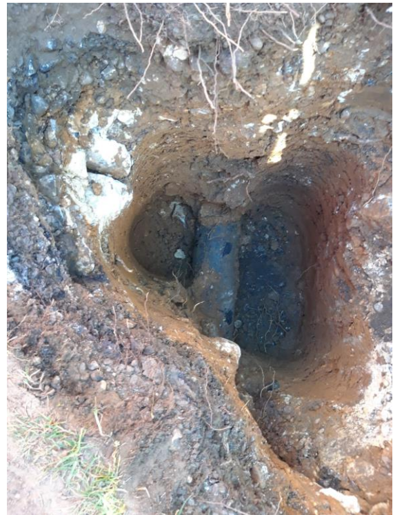
An example of a Utility Trial Hole
